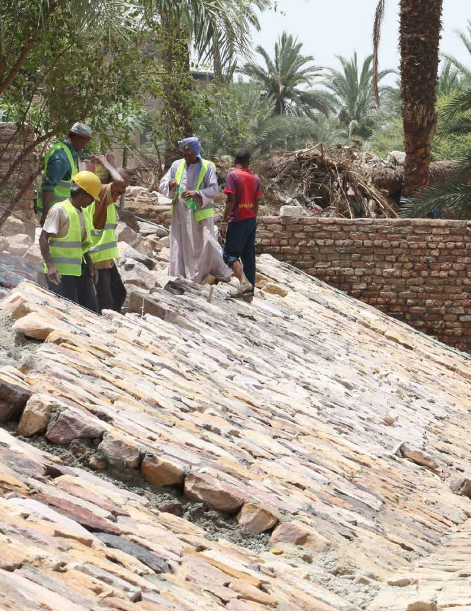
Construction workers in Luxor, Egypt, build stronger river banks along the Nile River. Photo credit: Dominic Chavez/World Bank.
